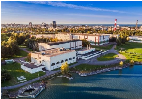
Ülemiste Water Treatment Plant
