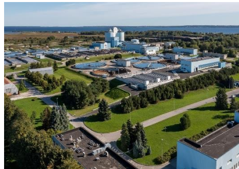
Paljassaare Wastewater Treatment Plant
