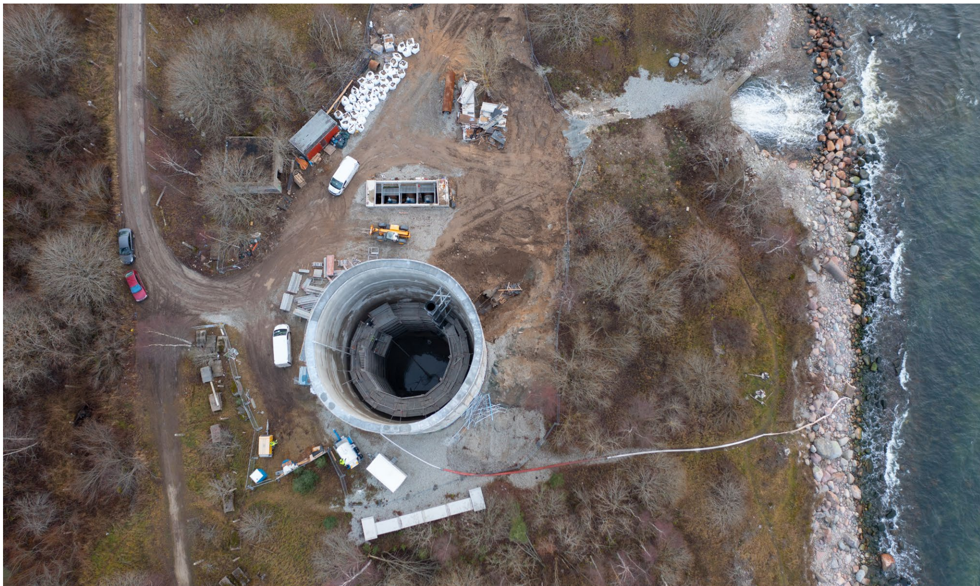
Reconstruction works of effluent outlet tower
